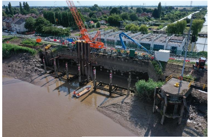
New outfall works
